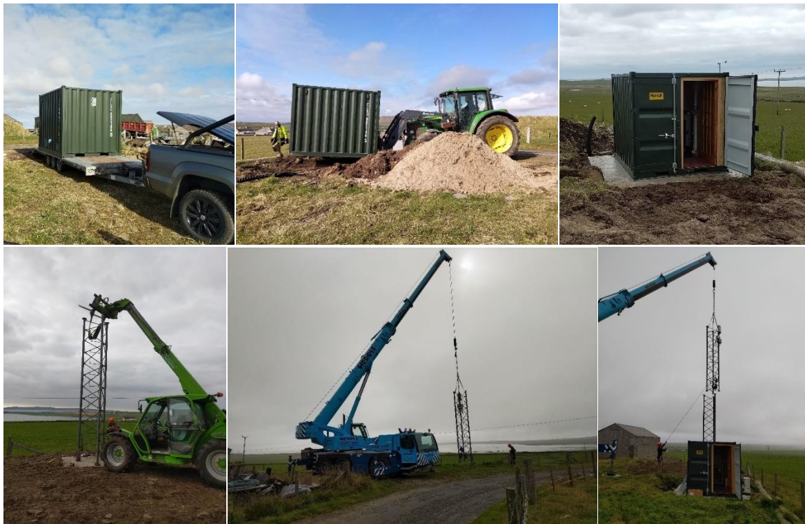
Figure 2.9: Installation of comms room and mast at Kirkbrae hub site.
