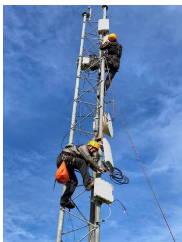
Figure 2.11: Radio equipment being fitted to towers.
