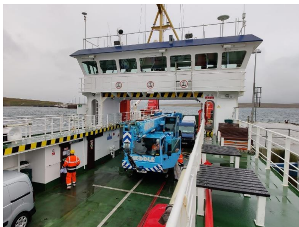
Figure 2.12: Crane on ferry for North Walls installation.
